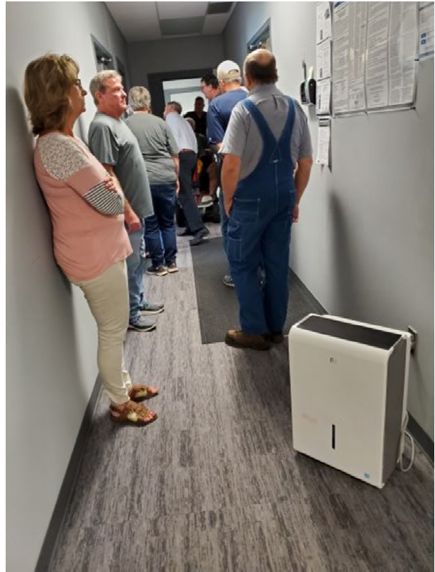
Figure #6. Supplemental dehumidification in the Administration area Corridor
