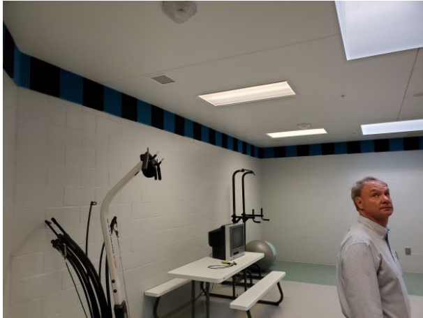
Figure #5. Indoor Rec area with Sky Lights and Sound-deadening material at the ceiling
